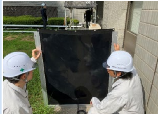
Film-type perovskite solar cells applying the construction methods under consideration
